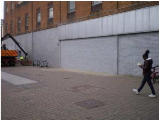
Moncrieff Place – the large windows (formerly Woolworths) have recently been removed and replaced with blank walls.
