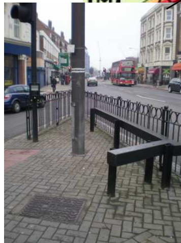
Cramped cluttered crossing pen for pedestrians.
