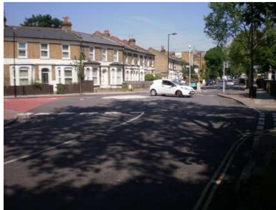
6.2 Pedestrian crossing distances increased significantly by large space taken up by mini-roundabout by Brimington Park - location of a number of collisions
