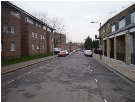
5.1 The introduction of greenery, removal of much unused carriageway and increased use by those on foot & on bikes could help bring streets like Godman Rd (above) and Bournemouth Rd to life.
