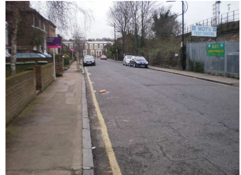
Blenheim Grove – looking west towards Bellenden Rd. Imbalance in the provision of carriageway space for vehicles and narrow and poorly maintained pavements.
