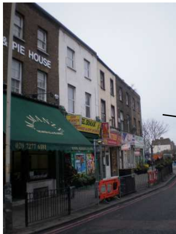
Narrow pavement – guard rail throughout.
