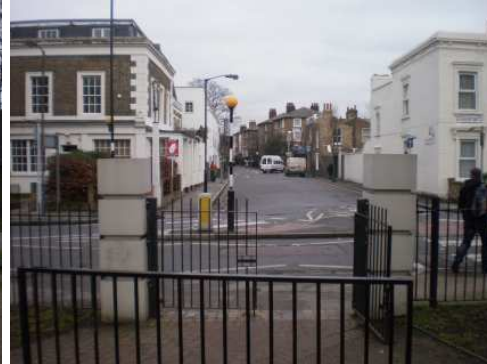
View east from Warwick Gardens – wide carriageway and extremely narrow pavements.
